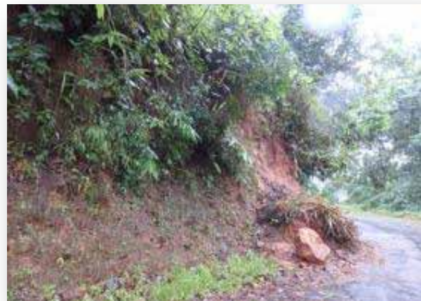
Photo: Road section at (km 13+000)
