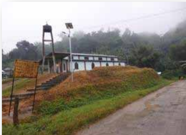
Photo: Road section at 20+851
