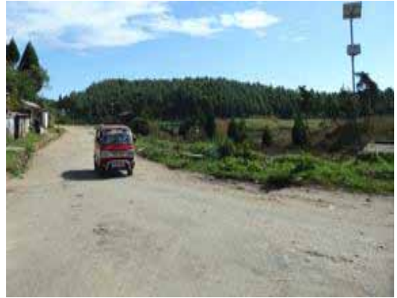
Photo: Road conditons at km 10+000
