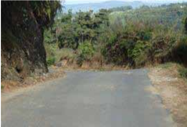
Photo: Road conditons& curve at km 6+10
